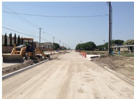
complete including meandering sidewalks, and the south bound lanes are approximately 95% complete. The contractor is constructing the medians and side street tie-ins. Remaining items to be completed include sidewalks along the south bound lanes, lighting and landscaping for the entire project. The newest section of Cockrell Hill Road will be consistent with the portion of Cockrell Hill Rd. that was completed from Belt Line Road to Wintergreen Road, thereby improving regional mobility.
